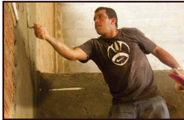
Pastor Ivanildo putting plaster on the walls
