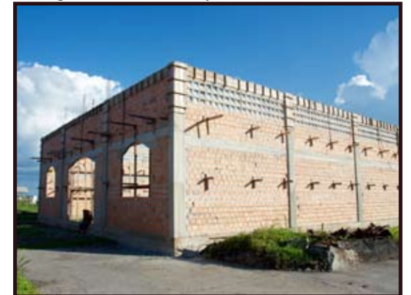
Construction of Portel Church
