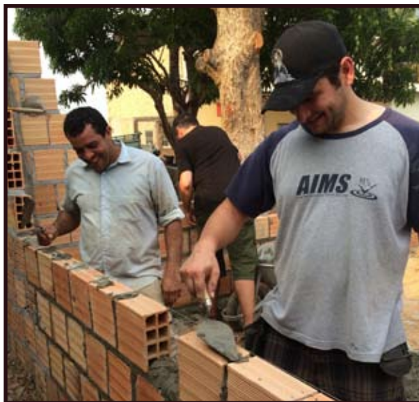
Laying the bricks for the Community Center
